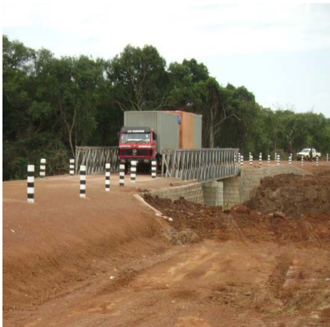
The refurbished Bandame Bridge, on the Yei-Maridi Road in Central Equatoria state. Photo: UNOPS
